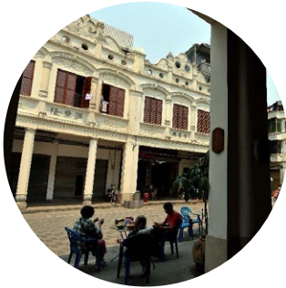
typology of Qilou- larger plinth and protection from heat and rain, Author: unknown, Retrieved from http://www.gd.xinhuanet.com/newsce-
