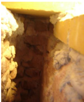
Figure 57 The cavity wall of BK City.
