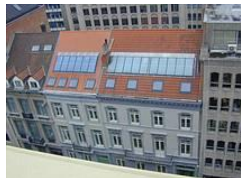
Figure 50 Solar Thermal collectors front façade, 'Renewable Energy House', Brussels
