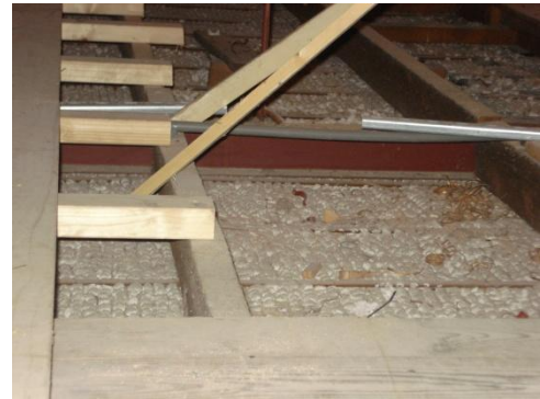
Figure 59 The existing rock wool insulation of the attic floor
