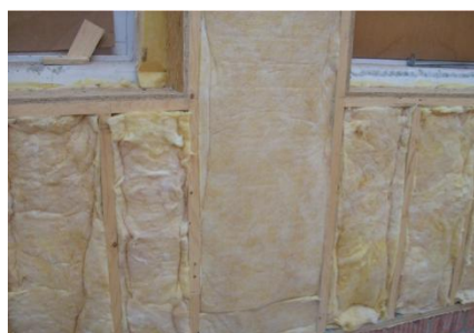
Figure 30 Details of the wooden framed inside wall insulation, 'Latijnse School'
