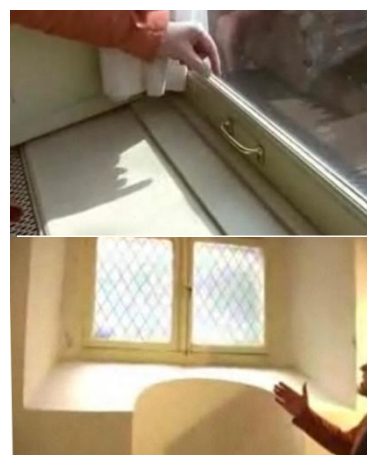
Figure 34 The narrow profiled existing windows favor the option of installing secondary windows (above). When that is not possible (below), the plan is to use thick curtains to minimize heat losses. ‘Paushuize’, Utrecht
