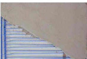
Figure 55 Heat and cold transport piping at the TUE campus, the Netherlands
