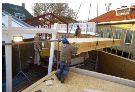
Figure 31 The steel structure for the roof support and the insulation elements, 'Latijnse School'
