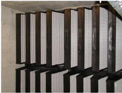
Figure 82 Example of a fine filter through which air will pass before entering the distribution chamber. The subsequent pressure loss could reach 50Pa
