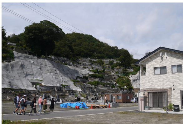
(a) Concrete slopes
