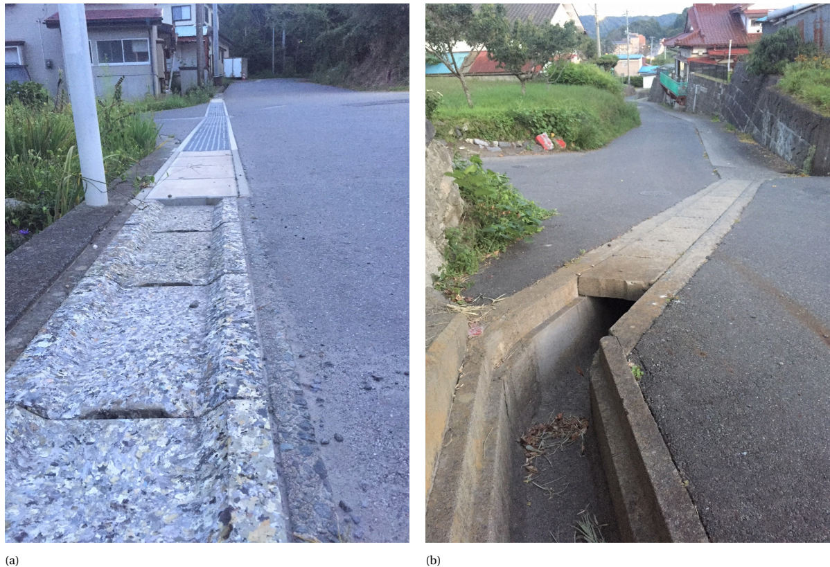
Figure 2.1: Examples of semi-open gutters to drain stormwater in Ōtsuchi town, Kirikiri district. Source: I. Nederlof
