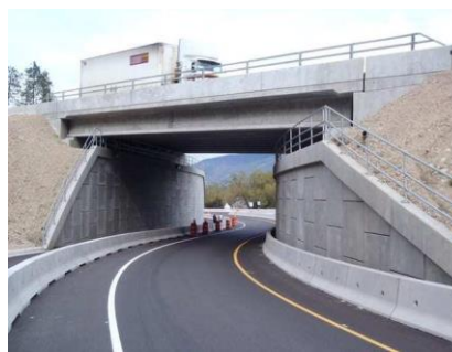
Figure 49: Curved wing walls
