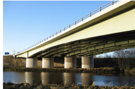
Figure 47: Varying girder height example
