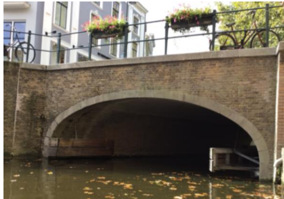
Figure 77: Arch bridge brick
