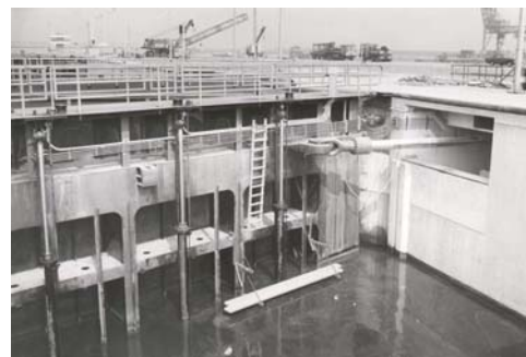
(b) Hydraulic cylinder gate operation mechanism of the mitre gates and sluices at Rozenburgse lock
