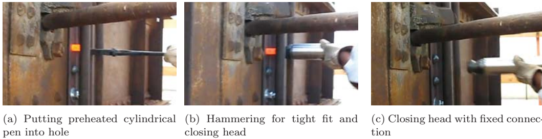
Figure 2.6: Fabrication of rivet joints [23]
