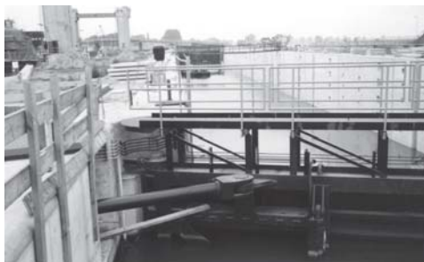
(a) Hydraulic cylinder gate operation mechanism of the 'Tweede sluis' at Lith
