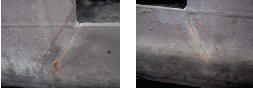
Figure 3.6: Cracks in horizontal and vertical girders
