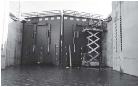
(a) Lock paddles for the rectangular openings of the 'Kleine sluis' in IJmuiden [14]
