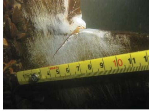
(b) Crack in horizontal girder [12]
