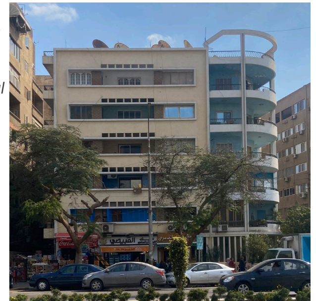
Figure 86 : Building B side view.
