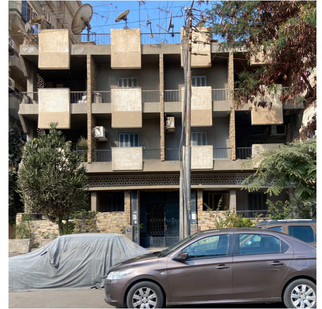
Figure 92 : Building D front view.
