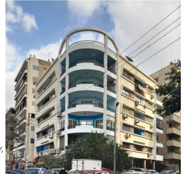
Figure 85 : Building B front view.
