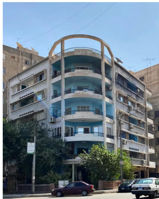
Figure 26: Discussion over restoring El Hegaz street architecture as a showcase for modernist architecture. 21
