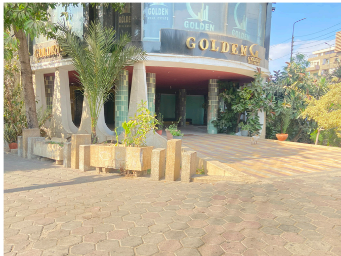
Figure 83 : Entrance of building A.
