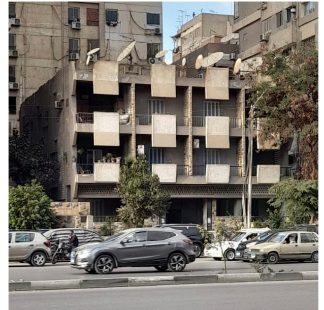
Figure 93 : Building D front view.
