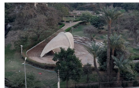
Figure 31: Example of a focal node highlighted by a concrete structure. 23
