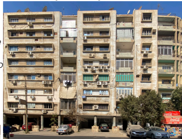
Figure 79 : Building A side view.
