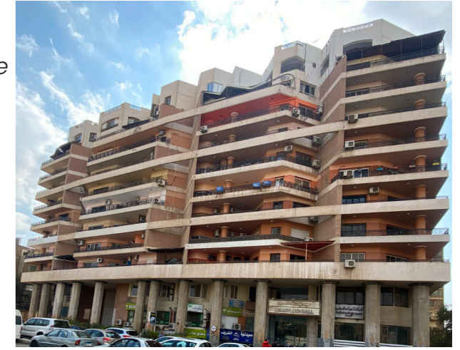
Figure 75 : Merryland mall building.
