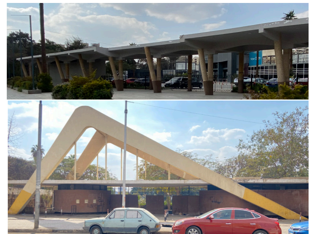
Figure 30: Images of the Merryland park entrances new at the top and old at the bottom
