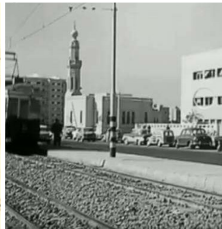
Figure 46: Image showing mosque in early stages. 34
