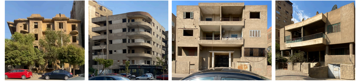
Figure 19: Images showing buildings that appear to be in the process of demolition currently in EL Hegaz street.
