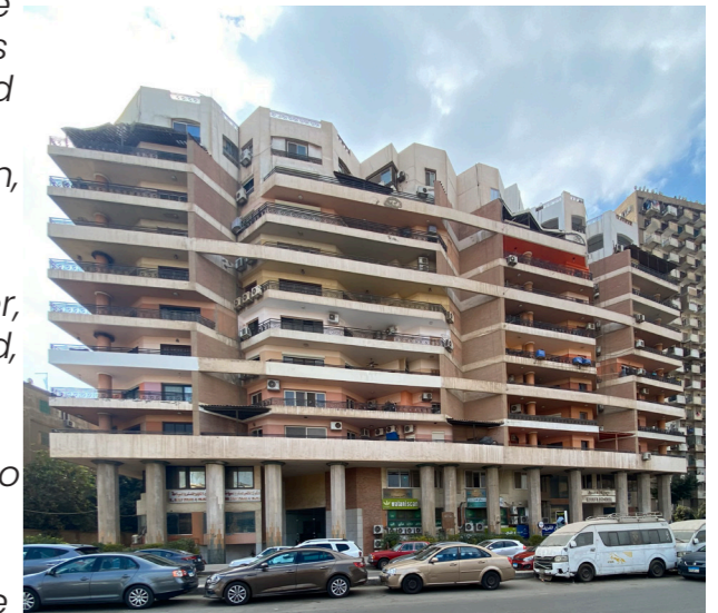
Figure 76 : Merryland mall building.
