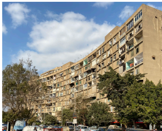
Figure 68: Image of curved building.
