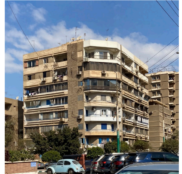
Figure 99 : Building G front view.
