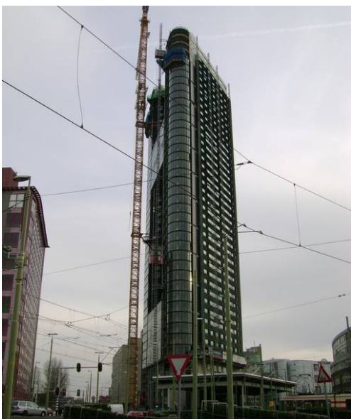
Figure 1-1: Strijkijzer, Den Haag. Tube structure composed of precast concrete elements
