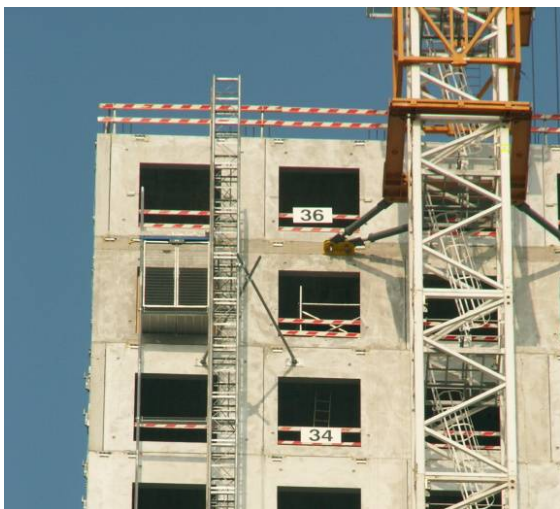
Figure 3-10: Staggered corner connection at Maastoren
