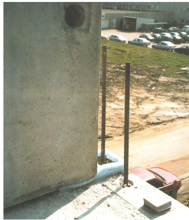
Figure 3-9: Preparations for precast corner connection
