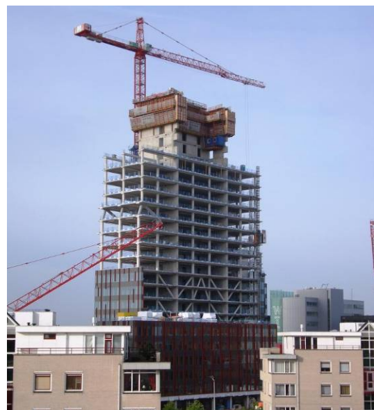
Figure 1-2: Carlton, Almere. Apart from the core all structural elements are prefabricated
