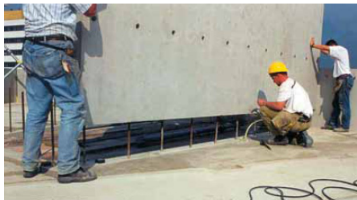
Figure 3-5: Lowering the upper element over the protruding bars (Handboek prefab beton)
