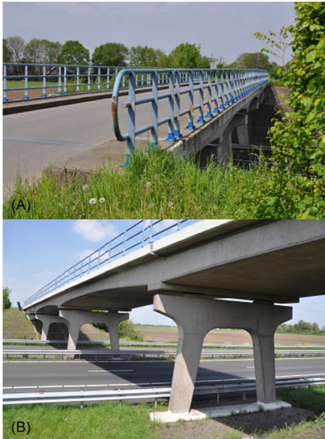
Figure 6.1 Photograph of viaduct Zijlweg: (A) top view; (B) bottom view.
