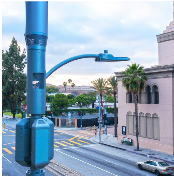
Figure 16 - Concealed 5g small cell on a light pole (Conceal-Fab, 2023).
