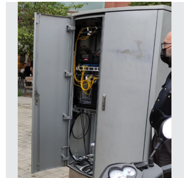
Figure 15 - Standard metal box edge equipment enclosure in Barcelona (Lenovo Press, n.d.).
