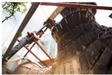
(b) Applying cement-paste coating
