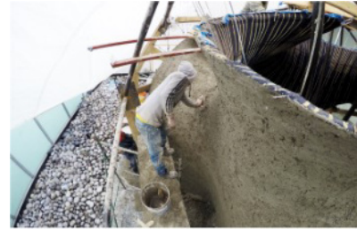
(c) Applying concrete
