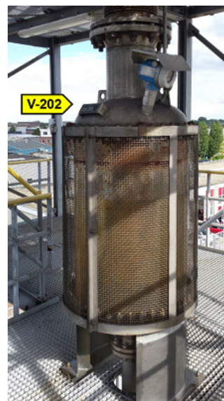
(b) Vessel V-202 serves as a temporary water storage tank upstream of the pump.
