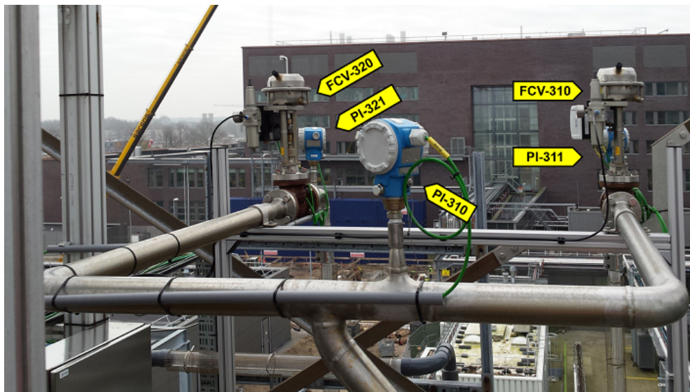
Figure B-9: Top section where the flow from both risers is combined.
