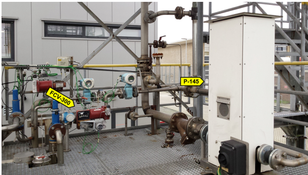
Figure B-1: Pump P-145 and control valve FCV-300 that regulates the liquid flow rate.
