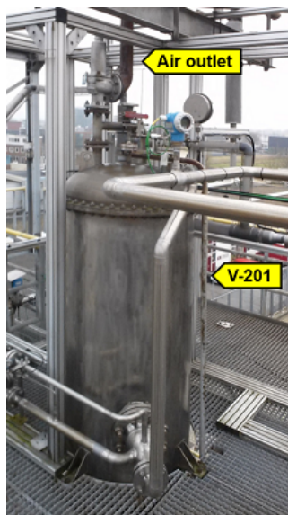
(a) Final pipe segment of the top section and separator vessel V-201. The air is released in the atmosphere and the water flows down into vessel V-202.
