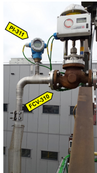
(b) Right riser head configuration with pressure indicator PI-311 followed by a choke valve FCV-310.
