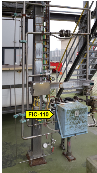
(a) Gas mass flow controller FIC-110 that extracts the air from the STCA air supply.
