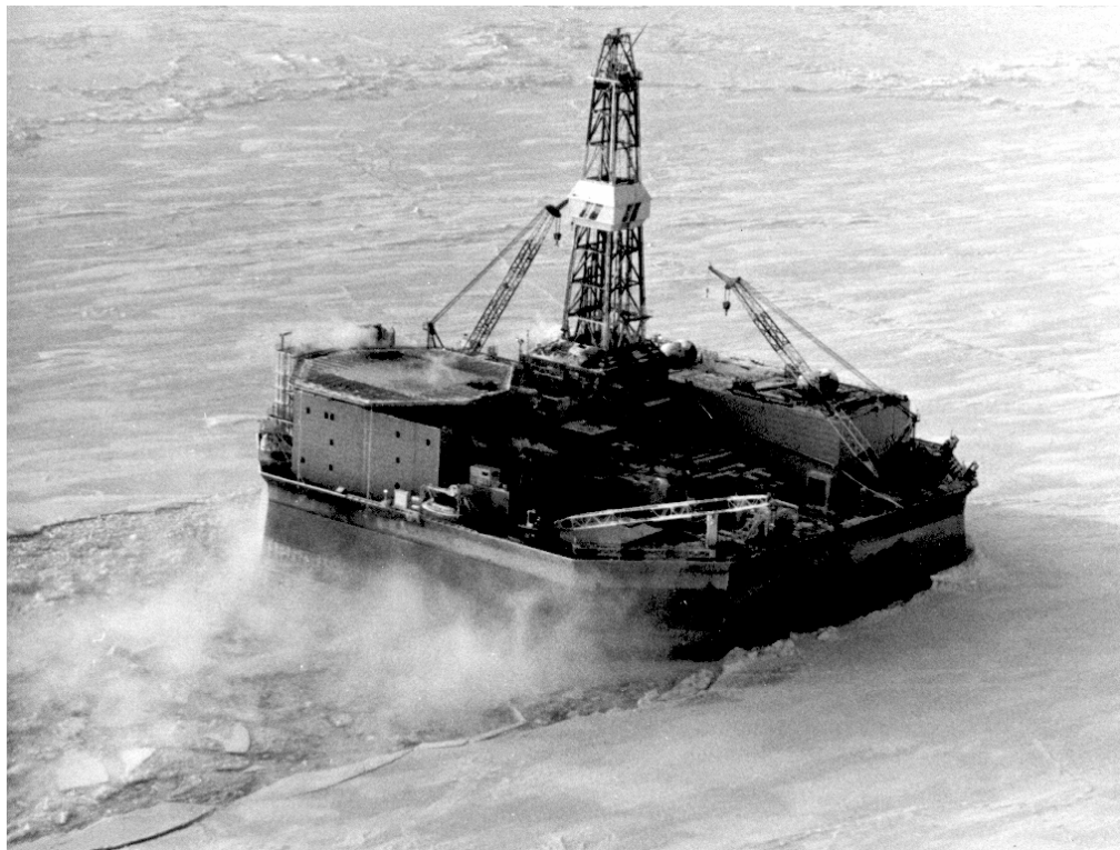
Figure 2. Photograph of Molikpaq in moving first year ice (note arrangement of short and long sides forming the octagonal plan)
