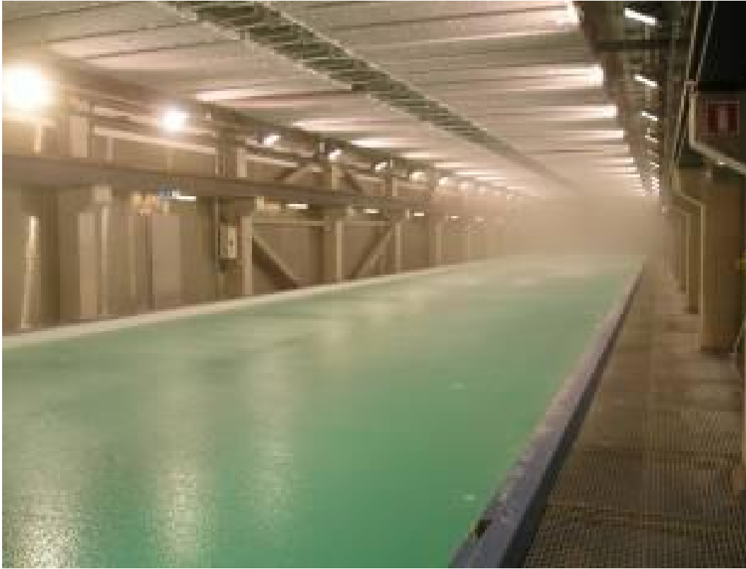
Figure 3. View to basin
