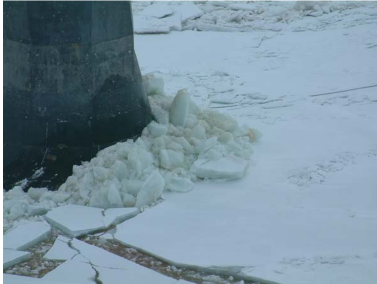
Figure 1. Typical ice Pile-Up on Confederation Bridge Pier
