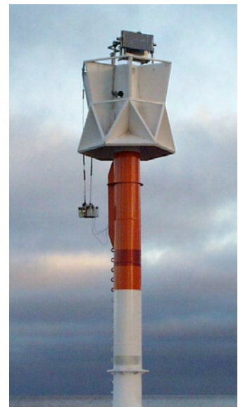
Figure 3. A modern channel edge marker superstructure.
