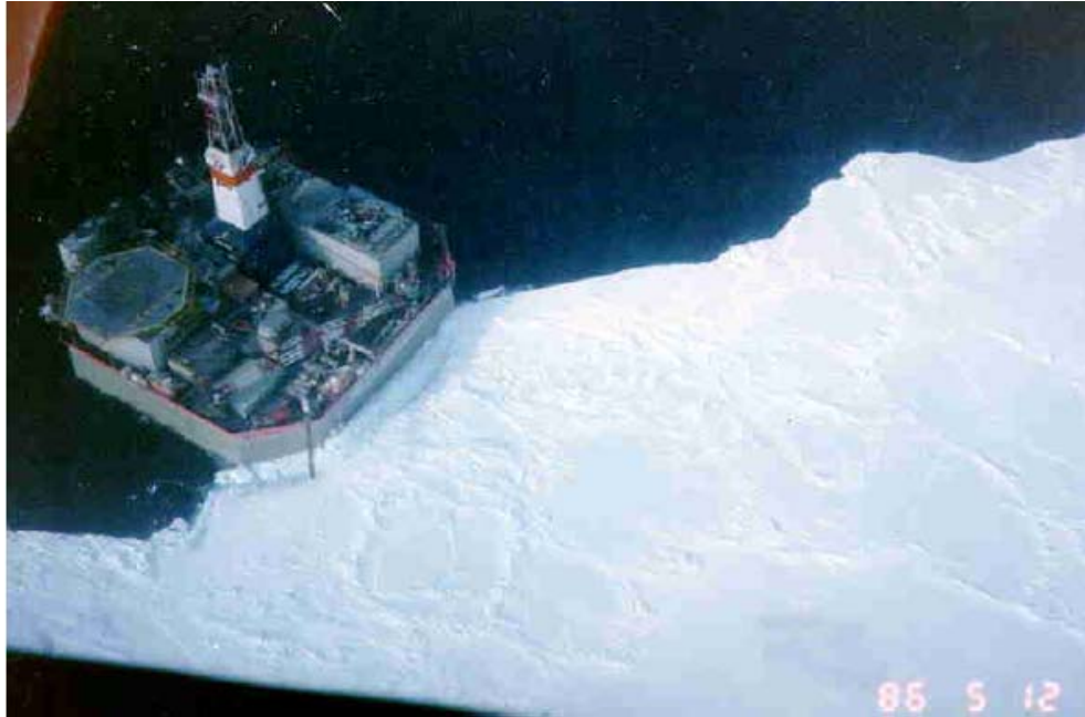
Figure 7. Aerial photograph of ice against north and northeast sides of Molikpaq after 12 May 86 event. The photograph was taken during the post-event helicopter ice reconnaissance flight by Volker Neth, P.Eng. (from GCRL project files). The ice had broken away from northwest side during the event and this area was in open water at the end.
