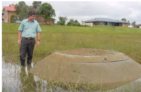
Figure 2.3: A sand boil around the exit on the land side of a dike [6]
