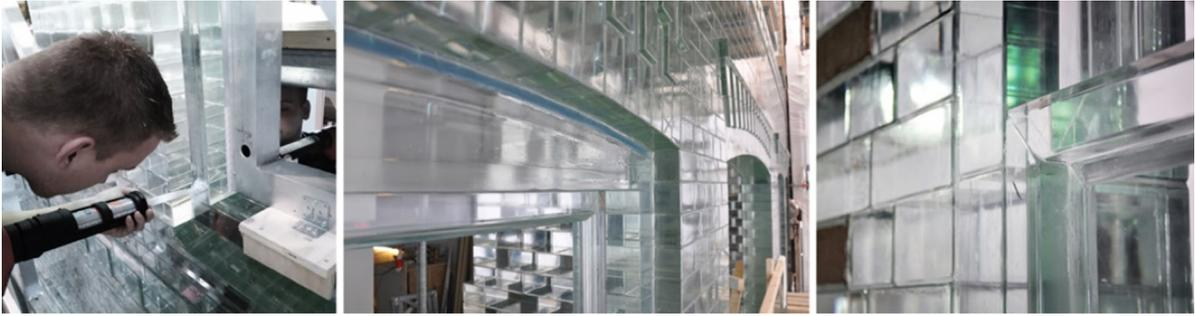
**Fig. 28** *Left:* The simultaneous application of the polymer from both sides. *Centre and right:* The final result of the bonded glass frames
