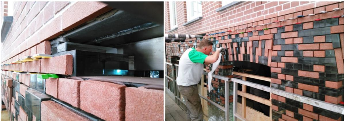
**Fig. 21** The *top connection* is completely masked by the ceramic strips
