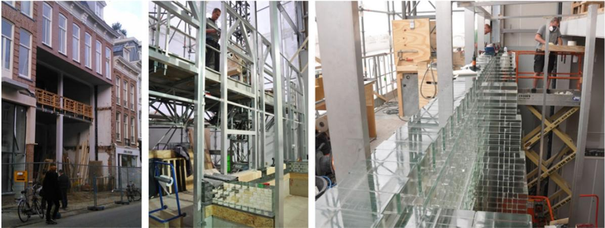
**Fig. 14** *Left:* The masonry wall was already constructed prior to the glass elevation. *Centre:* the installed aluminium place holders of the opening. *Right:* The mast climbing working platform and one of the three mobile elevated platforms
