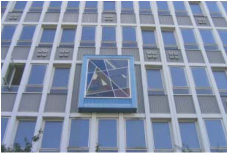
Figure 62: Characteristic pieces of art integrated in the building “Enka” were kept.
