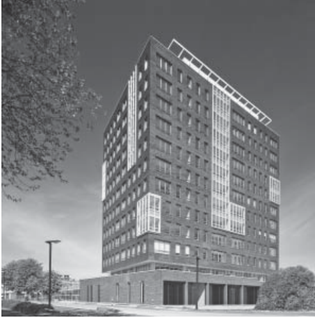
Figure 57: Twentec building, the facade was completely stripped and renewed. (Vesteda)
