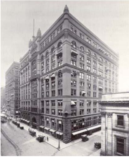
Figure 11 The Rookery building (Burnham and Root 1888). A transitional structure in modern architecture evolution, employing both masonry wall-bearing and skeletal frame construction techniques. (Bluestone, 1991)
