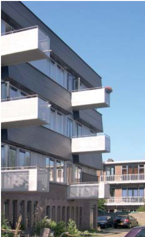
Figure 59: The 5,4m structural grid of the “Westplantsoen” was beneficial for transformation into student housing. The existing facade was upgraded. An additional floor was added on top of the building.
