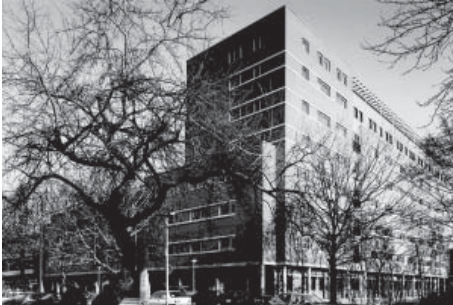
Figure 50 Two examples of transformations from offices into student housing, the GEB tower and the Bredestraat, both by Stadswonen in Rotterdam
