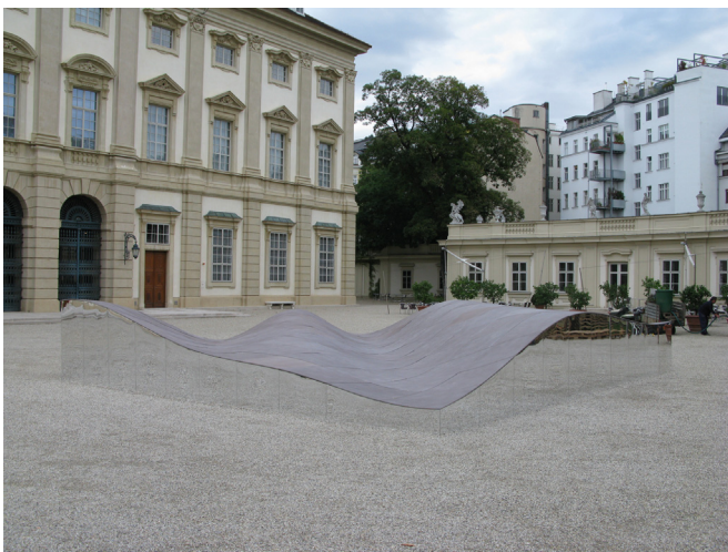
Fig. 6. Finished art project, where the GFRG elements has been cured on hot wire cut polystyrene.
