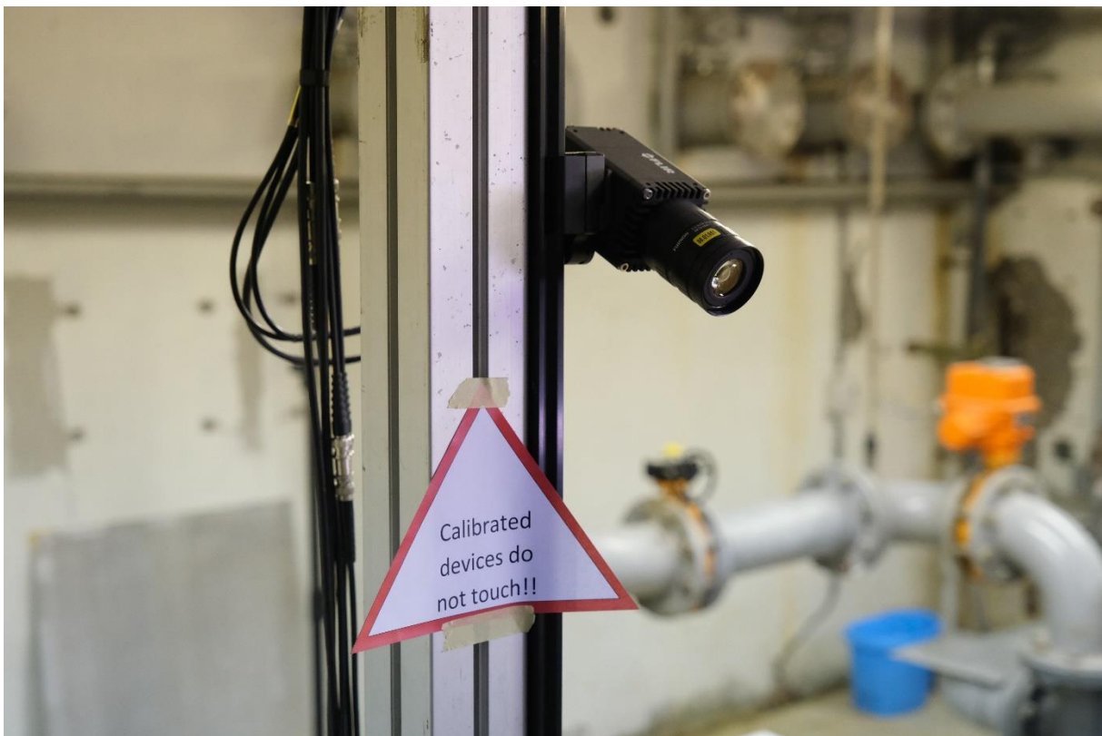
Figure 19 - One of three PTV cameras. After calibration, the cameras should not be moved even the slightest, hence the sign.
