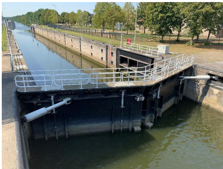
Figure 26 Set of mitre gates at the east side of the Marksluis (own photograph)
