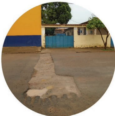
roads and the installation of the sewage system
