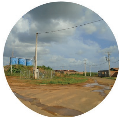
water reservoir in the neighborhoods
