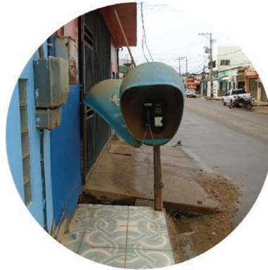
public telephone blocking sidewalk in one of the residential streets
