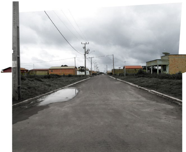
view of street in cidade nova (allotment development), single-family houses, spread out. very low density, little diversity
