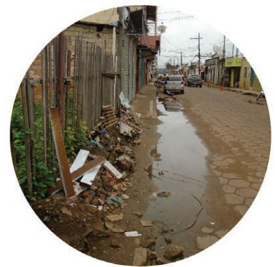
waste blocking the narrow sidewalk, poor drainage of the roads
