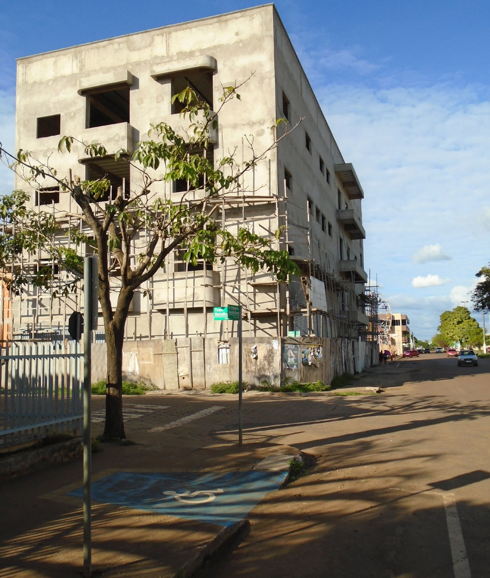
Figure 6.39 | Pluri-family housing project under construction photo by the author
