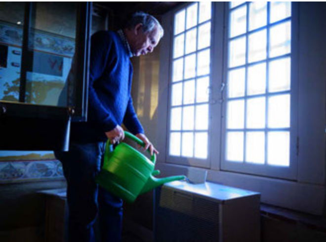
FIG. 3.1 A volunteer filling a humidifier: there is a risk of water being spilled / Photo Bart Ankersmit
