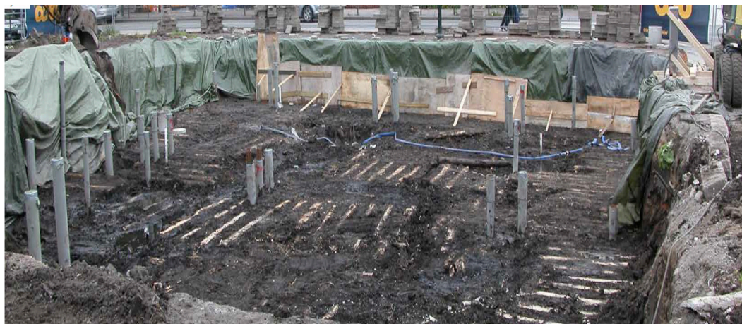
Figure 8: Archaeological deposits with monitoring devices J. Rytter.(2017). Piles drilled through archaeological deposits. Riksantikvaren.
