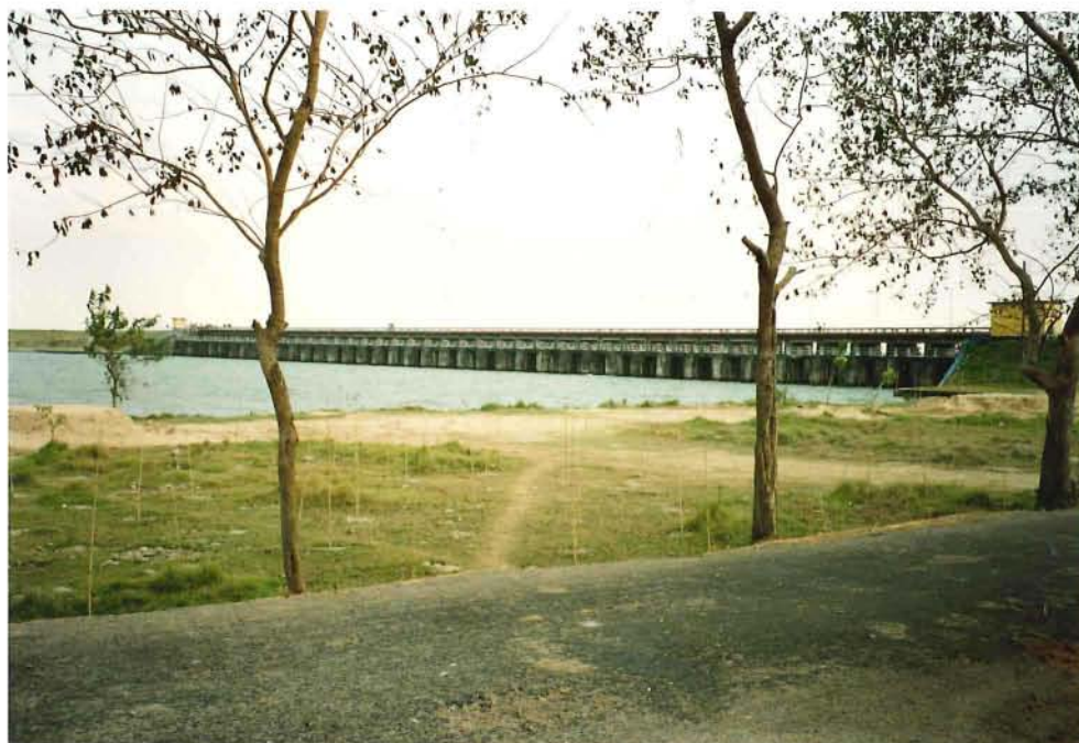
Photo 5: A complete view of the Regulator from the side of the approach channel. The radial gates are on this side, the flap gates on the other. One function of the Regulator is coastal defence: it is connected to the coastal embankment on both sides. Feni Dam starts on the left edge of the photo.
