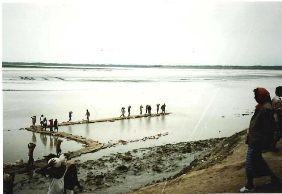
Photo 8: A groyne being built the Bengali way. This photo was taken at the eastern edge of the coastal embankment breach, near Sonagazi Regulator (see photo 1).
