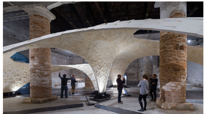
Figure 3. Thin Funicular Shell. Armadillo Vault. Block Research Group (2016).
