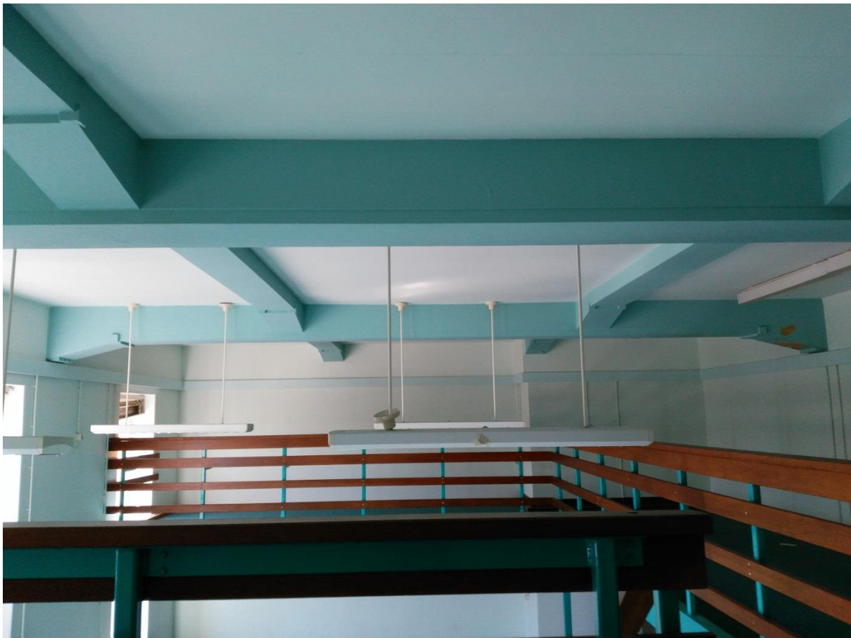
Figure 44 | The measured T-beams and cross beams in the old library section of the Maerlant
