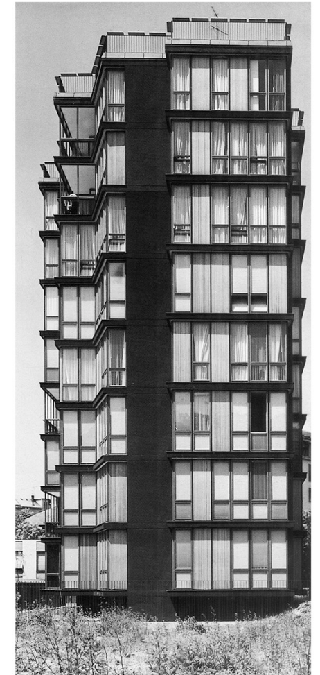
Prefabrication of wooden slatted panels, Via Quadronno, by architects Angelo Mangiarotti and Bruno Morassutti
