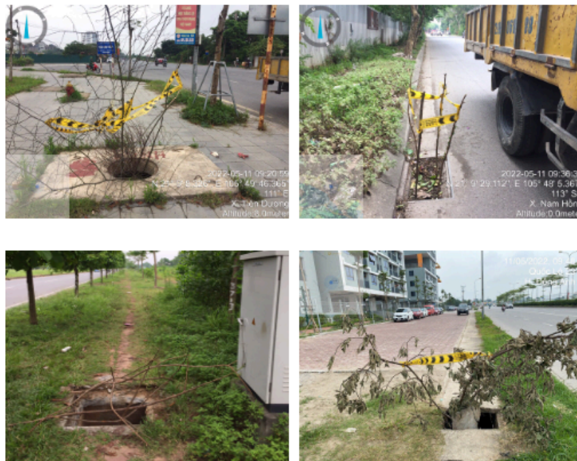
Figure B.2: Examples of drainage system components that are stolen. The drainage company places objects in the gap to prevent accidents. These objects block practically block flow through the pipeline. Source: Hanoi's drainage company, pictures taken by Nguyen Trong Nam
