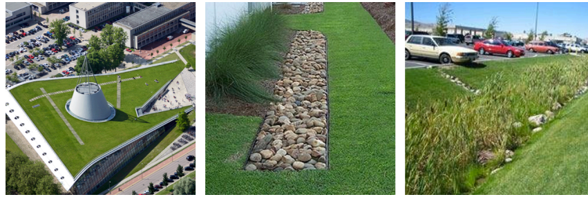
Figure 3.3: Examples of LIDs. Left: green roof, placed on top of the TU Delft University Library. Center: infiltration trench, right: vegetative swale. Source: Gambaro et al., 2012
