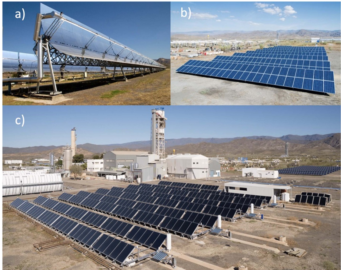
Figure 3. (a) PTC in operation, i.e. a parabolic trough collector used for CSP production. (b) A field of solar PV collectors. (c) A view of a field of stationary flat plate solar collectors that can supply heat at 80 °C.
