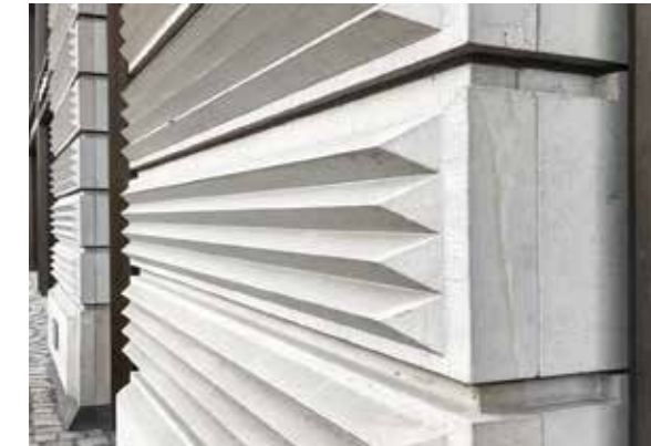
Fig. 12 Heavily textured surface of a suspended stone element
