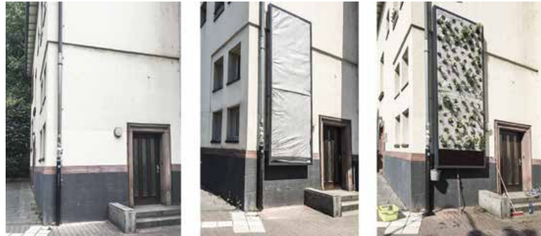
Fig. 10 a) Existing building b) Installation of substrate surface c) Green facade with fresh vegetation
