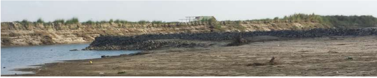
Figure 1.3: Bypassed barrier after a shift of a channel in the braided river the Ayeyarwady (January, 2017)
