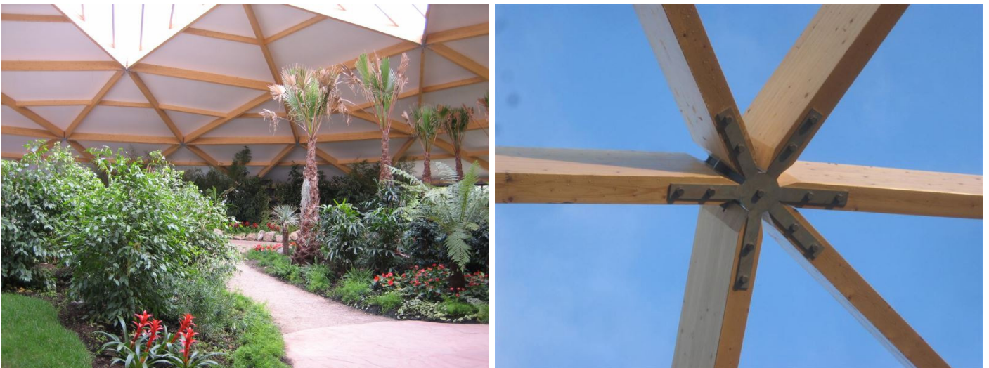
Figure 16 - Timber dome canopy, the Jungledome, Remouchamps (Lüning, 2006)
