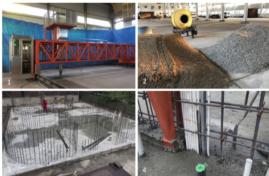
Fig. 2.23 On-site 3D-printing by HuaShang Tengda: 1. gantry-based printer with a hopper on the top of the printhead; 2. raw materials and mixer; 3. foundation and connective steel bars; 4. deposition of the first layer
