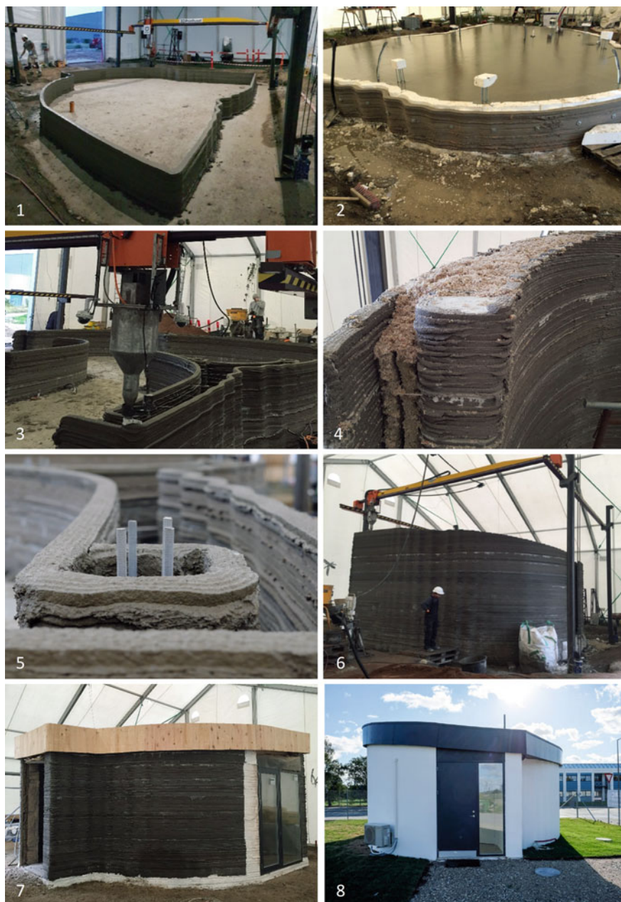
Fig. 2.11 Main phases in the construction of the BOD: 1. 3DCP of the foundation slab contour; 2. Concrete casting of the foundation slab; 3. 3DCP of the building walls and printing nozzle; 4. Detail of the insulation material; 5. Detail of the manually added rebars; 6. The BOD walls right after printing; 7. Application of roof, doors and windows; 8. The BOD after its completion
