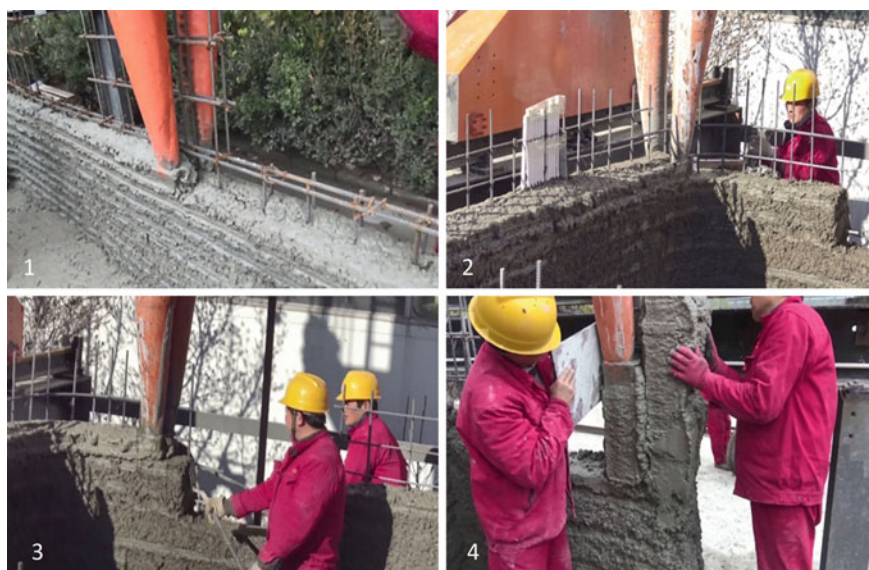
Fig. 2.24 Construction of the two-storey villa: 1. forked nozzle lays concrete on both sides of the rebars, 2. printing a bow; 3. manual help at the opening, when the material flow is interrupted; 4. forming a vertical element
