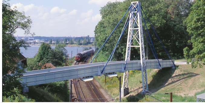
Figure 1.2: Fiberline FRP bridge in Kolding, Denmark Source: fiberline.com
