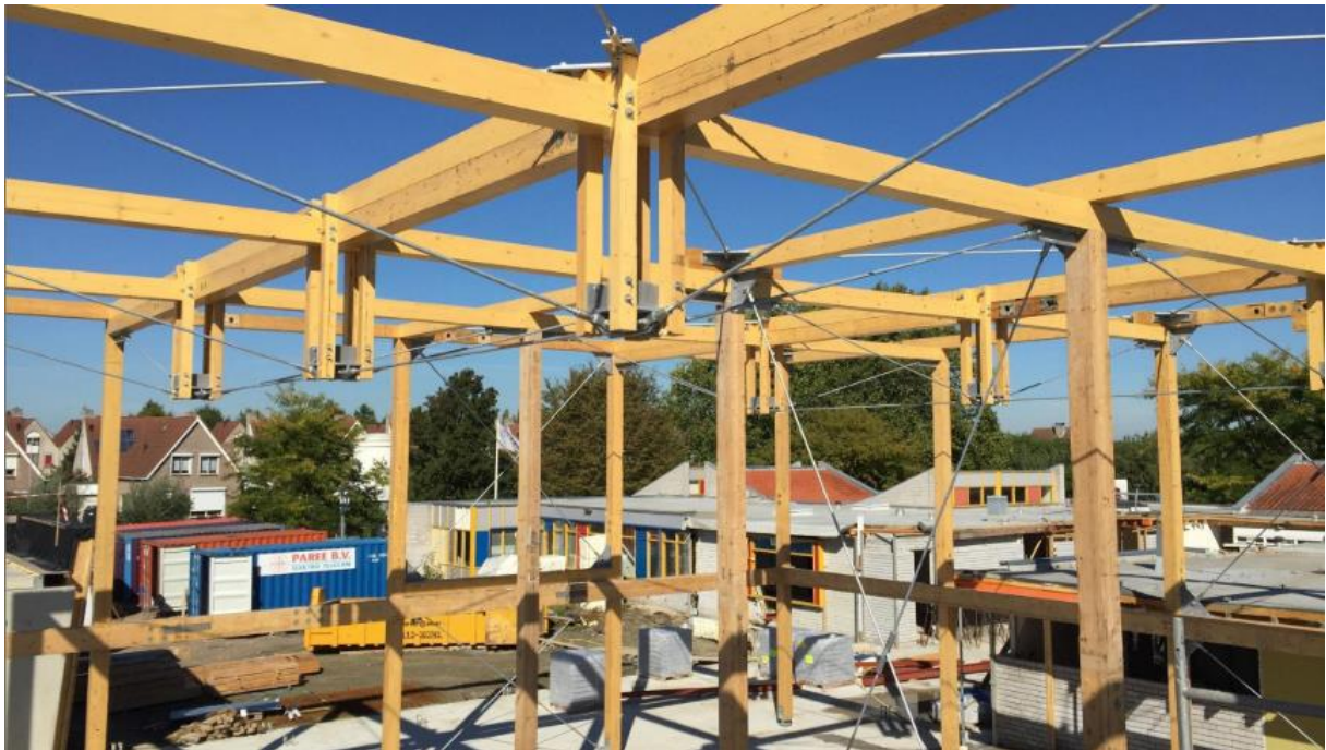
Figure 3.4.3 Construction of the Emergis-Ihtaka using the timber structure from Rijkswaterstaat in Terneuzen, Source: (B.v., n.d.)
