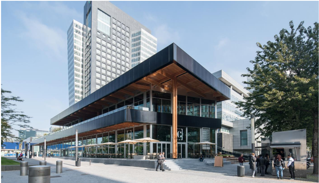
Figure 3.1.1 Exterior view of Circl Pavilion, Amsterdam, Source: (Cie, 2019)
