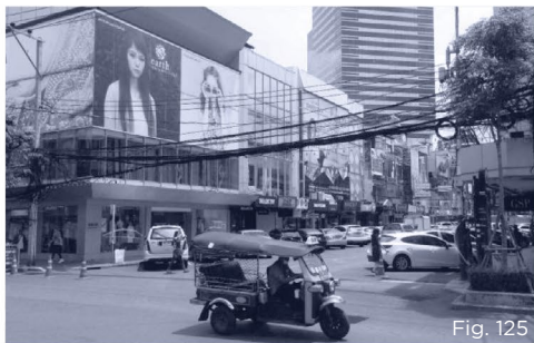
Low-rise Commercial : Siam Square Complex
