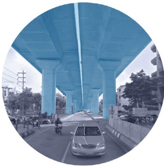
Lack of ecology system with unfriendly environment of highway structure
