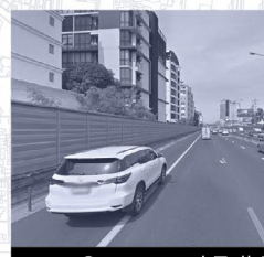
On-ground Toll Road (disconnect from surface)
