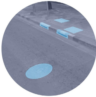
Underground drainage of mixed sewage and run-off
