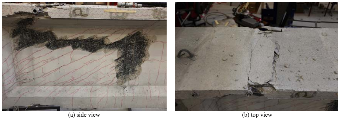
Fig. 15. Failure of beam 401 (first test)
