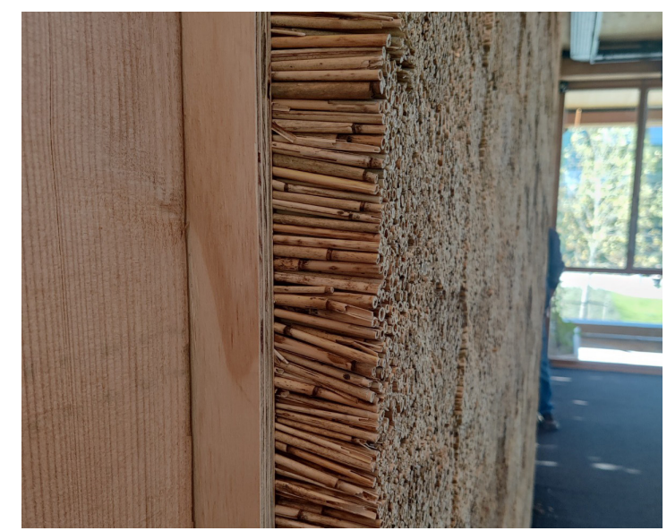
Reed/Straw insulation: -128 kg CO 2 / m 3 equivalent Stone wool 70 CO 2 / m 3 equivalent
