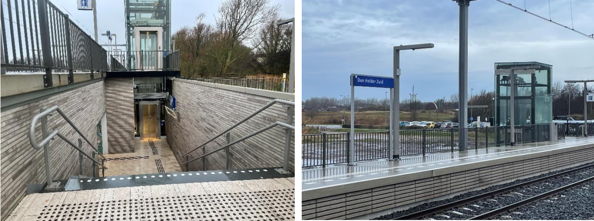
Figure 8. Pictures of Den Helder Zuid Station
