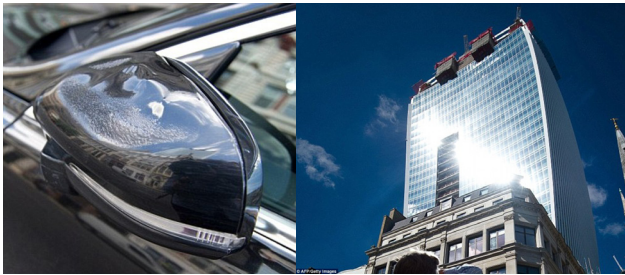
Figure 11.4.1: Damages caused by reflection of Walki Talki curtain wall facade .
