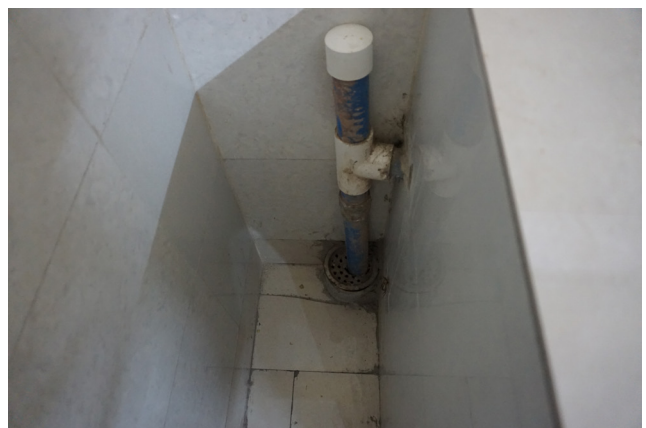
Figure 18: The drain in hospital 2.
