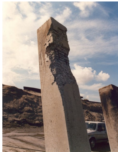
Figure 9. Pile damage.
