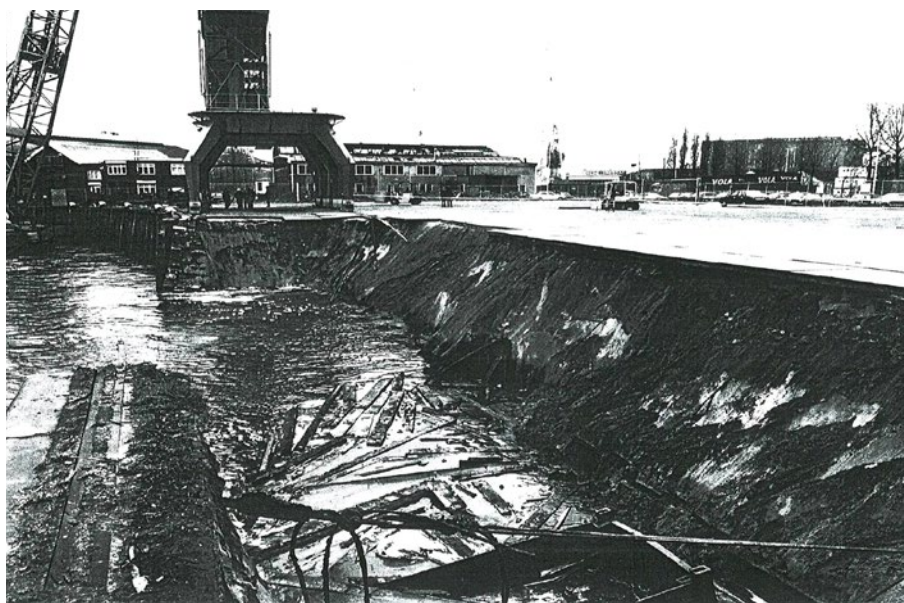
Figure 4. Failed quay wall Katendrecht.
