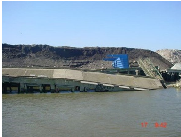
Figure 5. Failed jetty.
