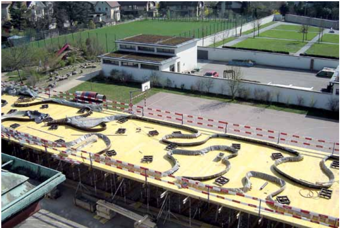
IV Christ & Gantenbein, Formwork on site, roof for a schoolyard, Muttenz, Switzerland
