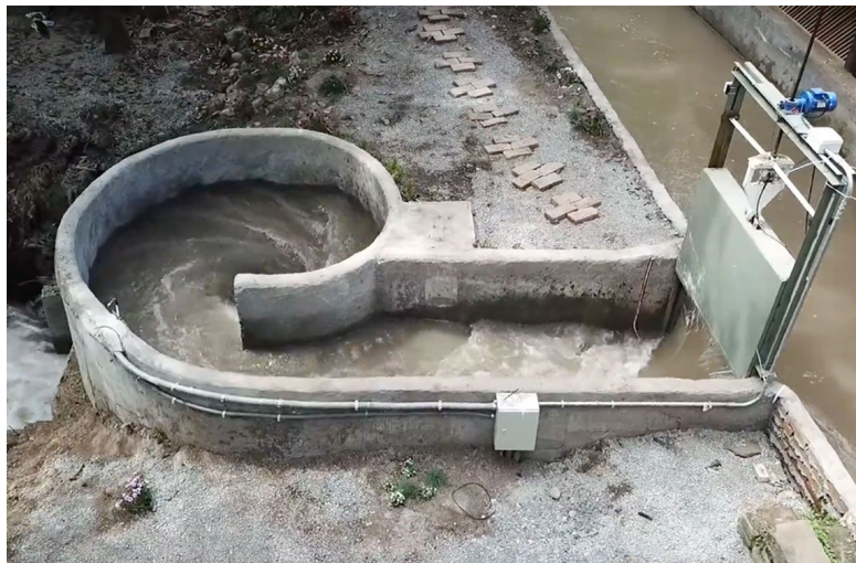
Figure 1: A 15 kW Turbulent turbine
