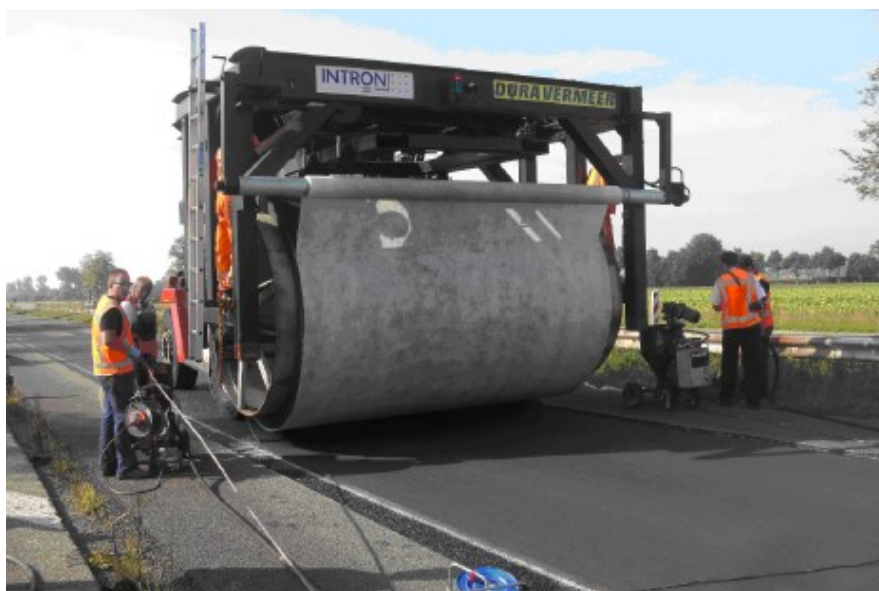
Figure 1. Construction of PERS road in Kloosterzande using Rollpave technique
