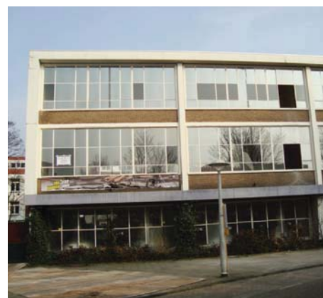
Figure 3.10: Primary school/community center (1954)
