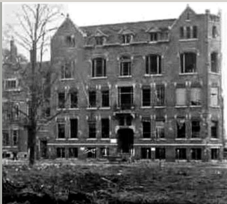
The former headquarters of the 'Sicherheits Dienst (SD)', at the Heemraadssingel in Rotterdam
