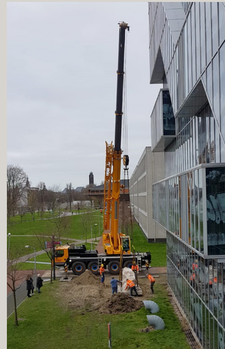
Installing the artwork in front of the faculty of Civil Engineering and Geosciences
