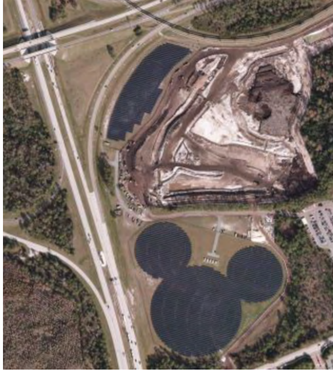
09 - Under construction / unknown
