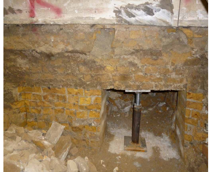
FIG. 3.11 Huis Nolet, basement: temporary support of the wall during insertion of concrete floor (December 2016) / Photo: B. L.ubelli
