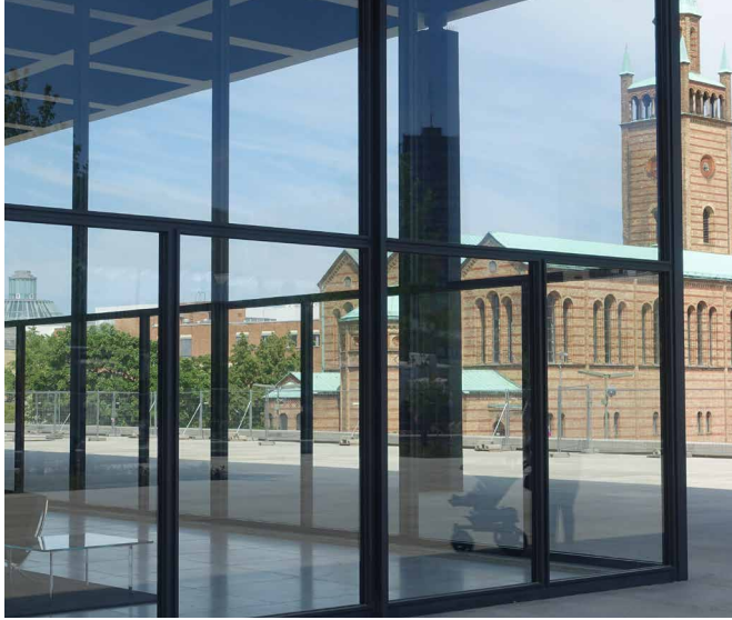
FIG. 5.39 New National Gallery, Berlin: original glazing (above) and three variants for the rehabilitation. In order to avoid glass breakage in the future, a double-thick laminated safety glass (2 x 12 mm) was used (second variant from above). The other two variants would have distorted the appearance of the construction too much. / Photo: F. May
