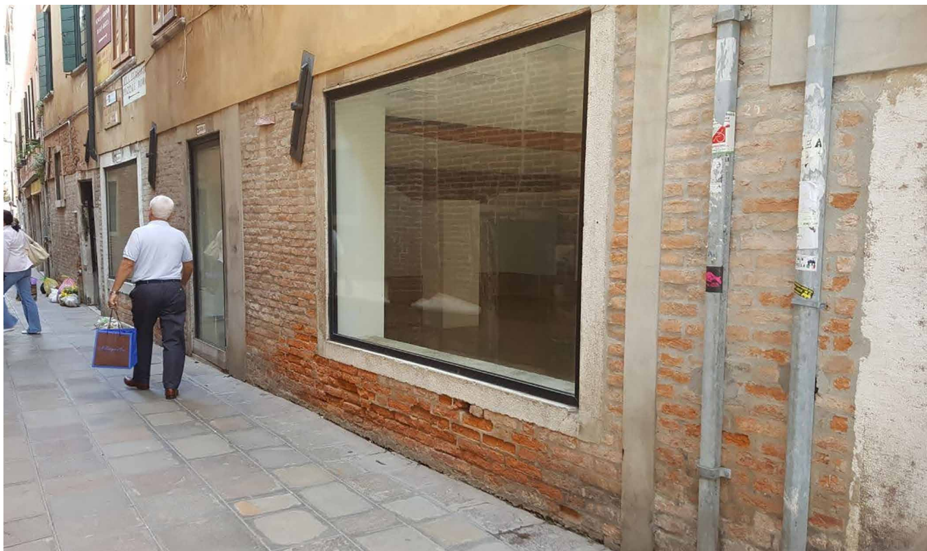
FIG. 3.1 Salt crystallization damage due to the presence of salts and rising damp, Venice, Italy / Photo: B. Lubelli
