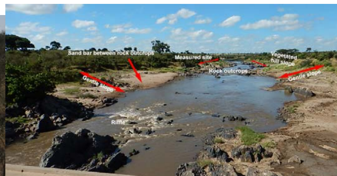
(g) River bed at Mara Purungat Bridge, from bridge looking downstream
