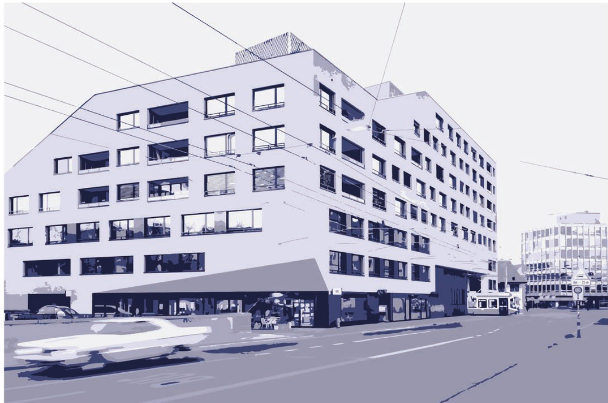
Figure 25. Edited by Author, Kalkbreite - Exterior View from the south.
