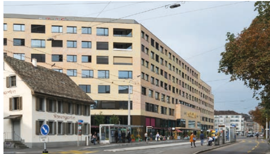
Figure 42. Kalkbreite - Exterior View (Rosengarten square).
