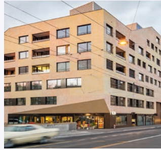
Figure 75. Commerce on the Ground Floor.
