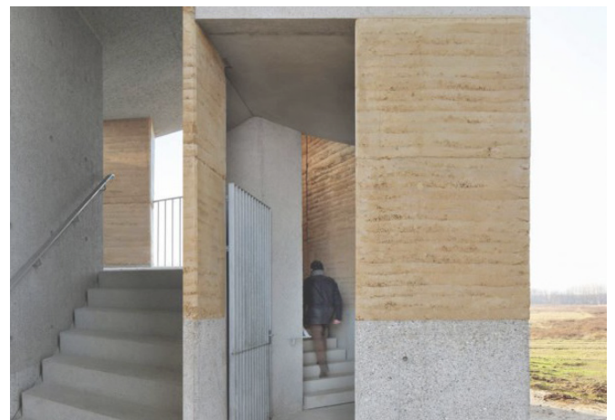
Figure G.9. Rammed-earth walls - Observation Tower by De Gouden Liniaal Architecte
